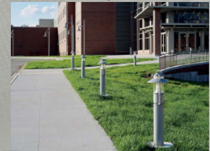
Either bollards or pole mounted fixtures for pathway and area lighting of plaza
